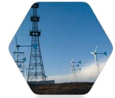
Telecom Base Station
